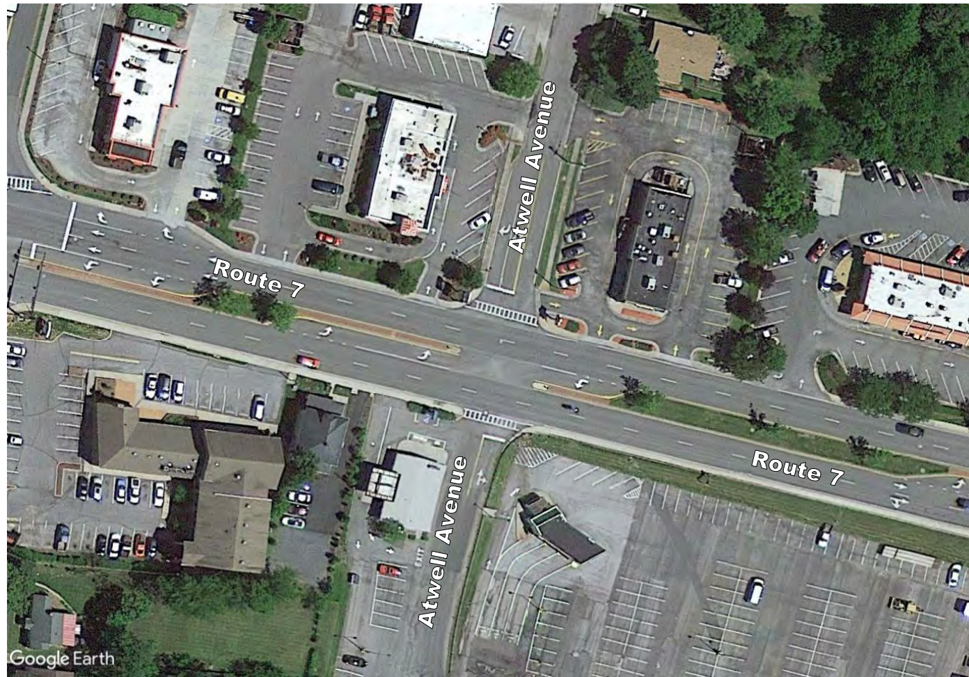
Figure 11: Route 7 at Atwell Avenue
