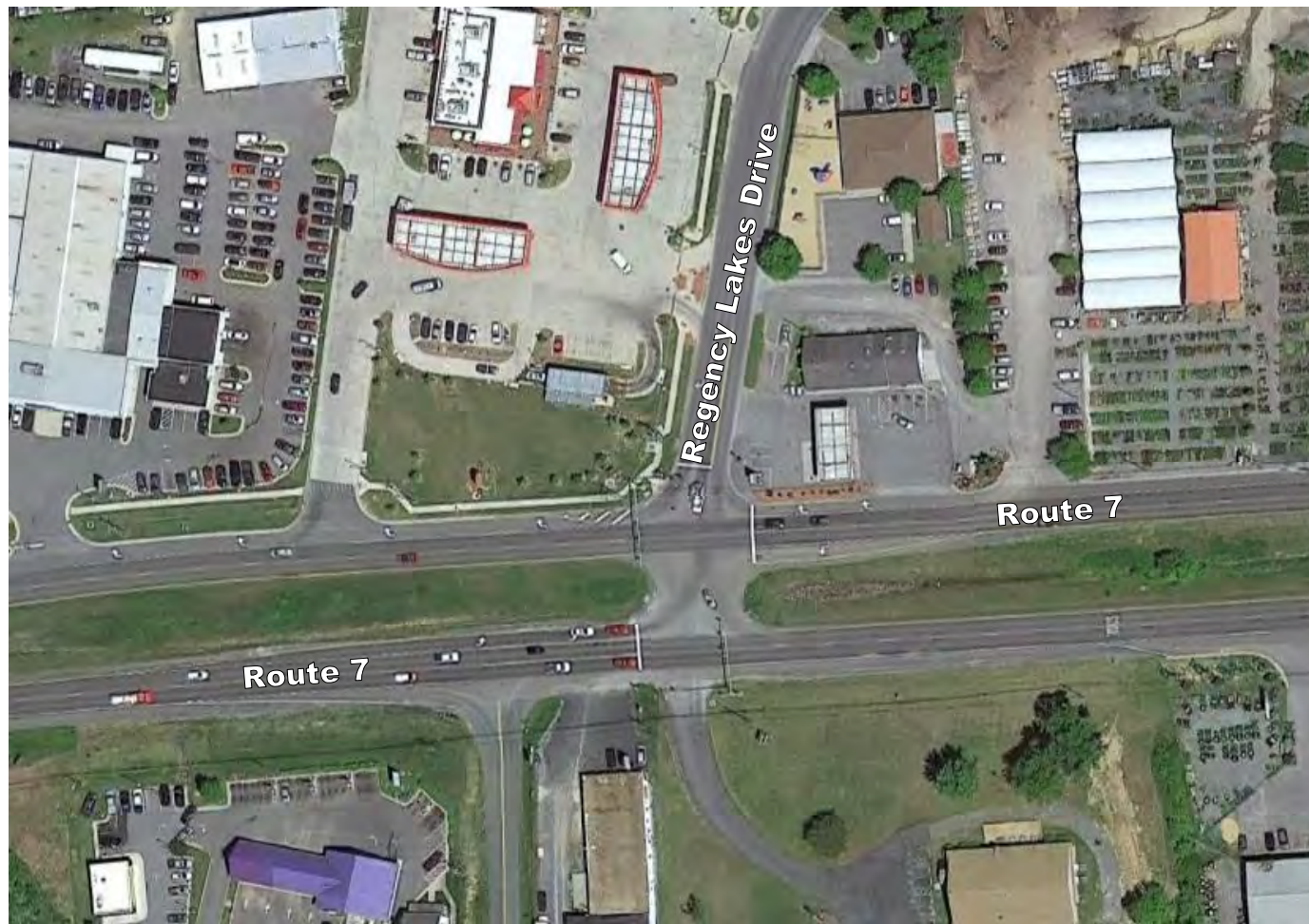
Figure 17: Route 7 at Regency Lakes Drive
