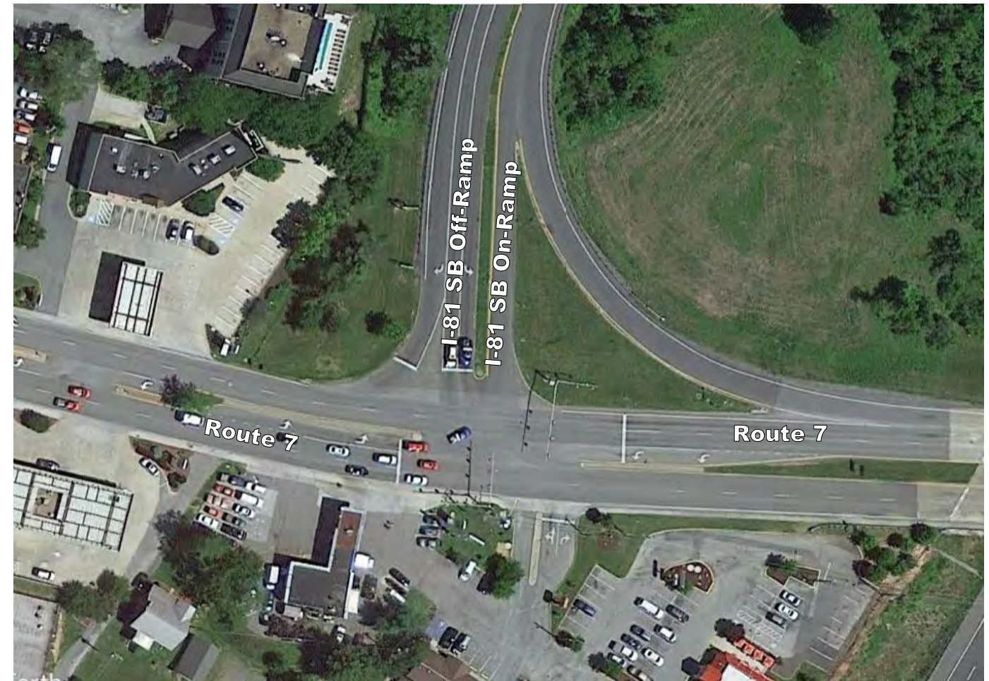
Figure 14: Route 7 at I-81 Southbound Ramps
