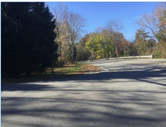
Figure 7.22c – View of NB Approach Sight Distance
