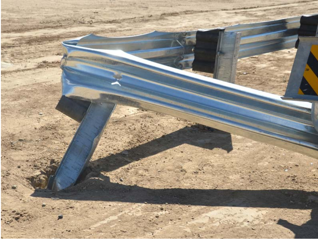
FIGURE 39. Test Article Damage
