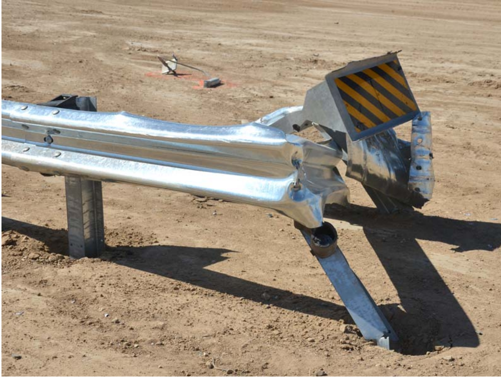
FIGURE 35. Test Article Damage
