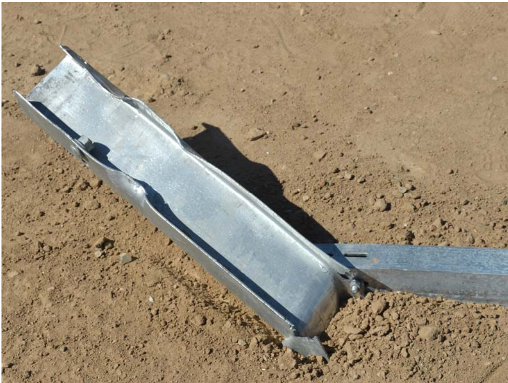
FIGURE 36. Test Article Damage
