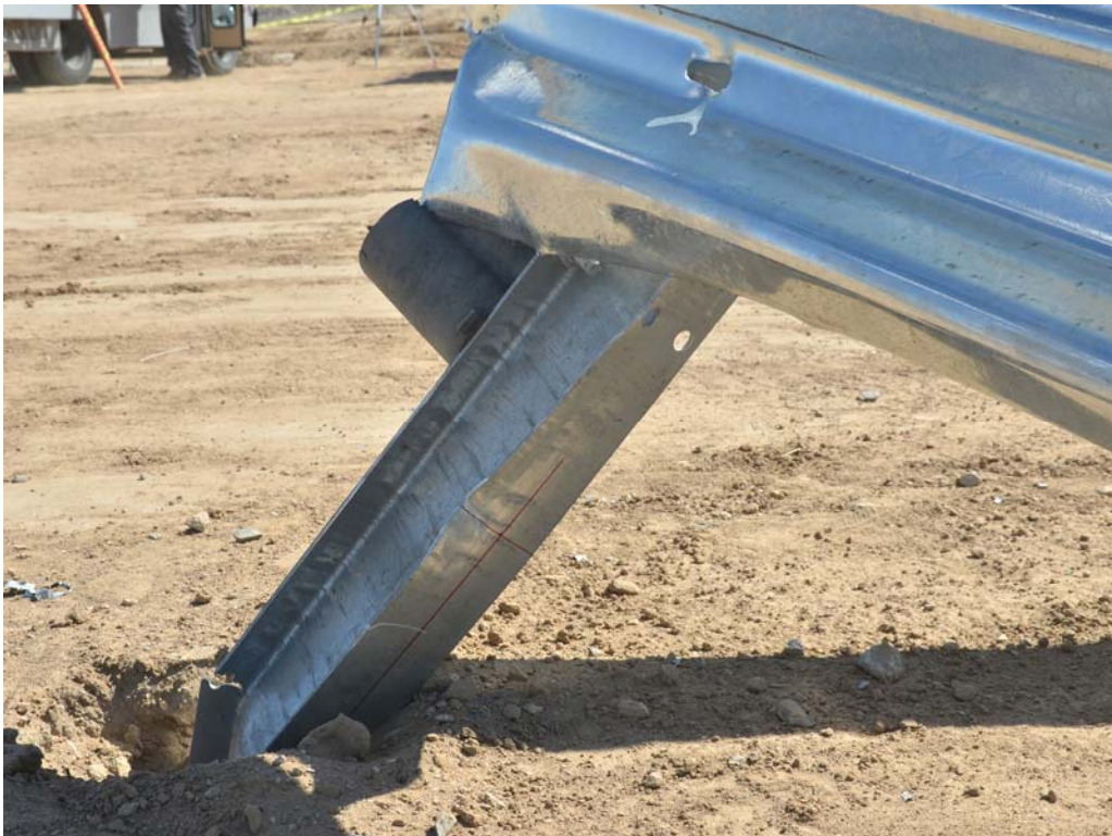
FIGURE 38. Test Article Damage
