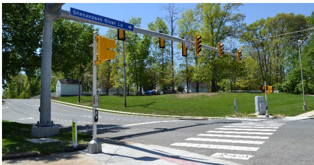
Improvements for pedestrian crossings on Shenandoah River Lane, Virginia.
