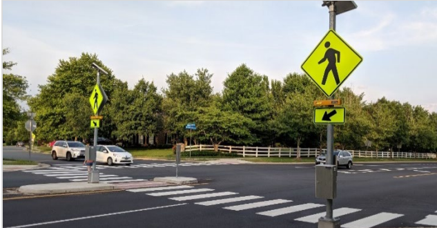
High visibility crosswalk with RRFB and median refuge island.
