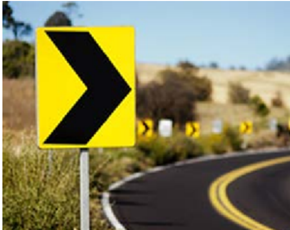
Chevron signs on the outside of a curve
