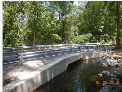
Photo: New bridge on Route 634 (Highgate Road) over Chippokes Creek
